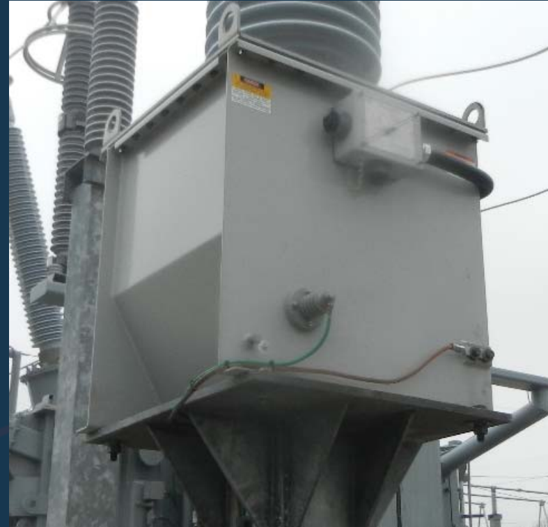
Properly Grounded H0 Connection
