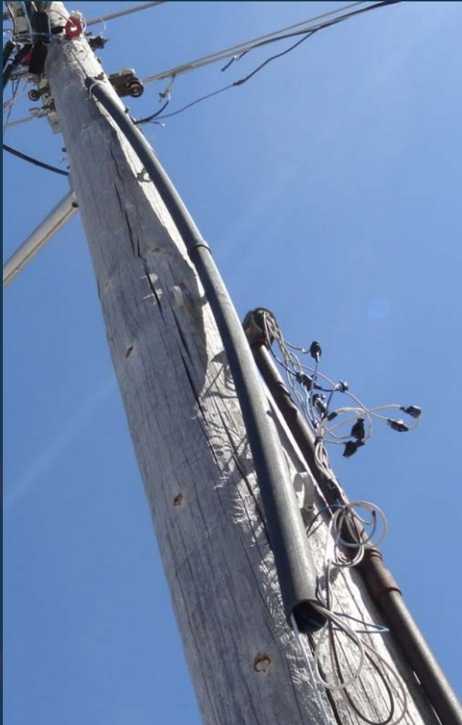
W T F : Wiring Total Fail !
