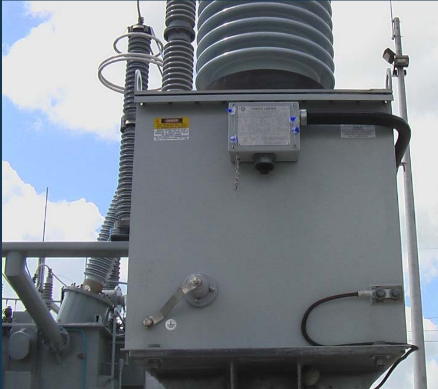
Improperly Grounded H0 Connection
