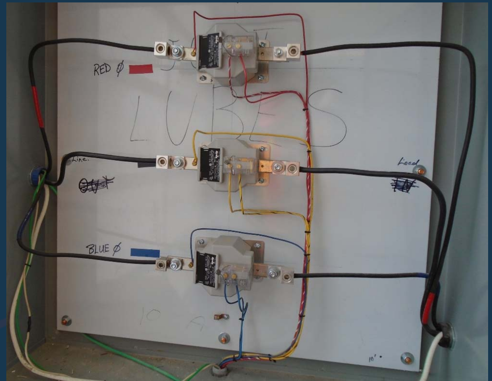
Not Grounded, CT's not Taped & 600V at Test Block / Meter
