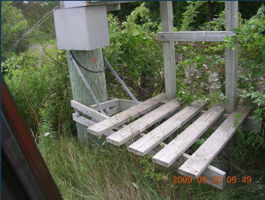
Broken & Unsafe Platform
