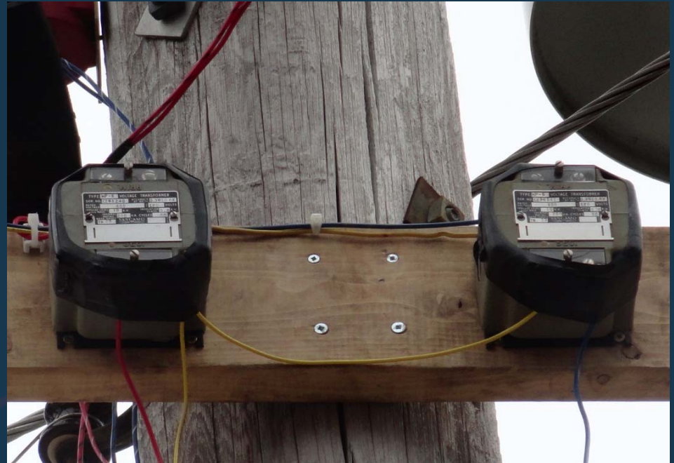
Indoor PT's at top of the pole
