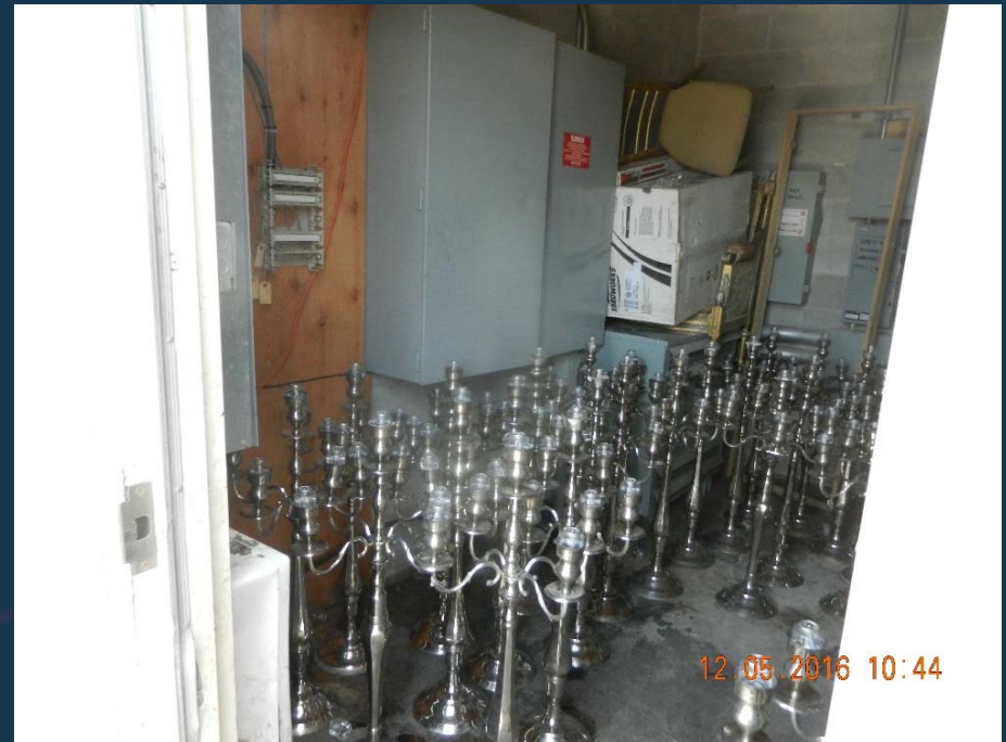
Improper storage space... Candles?
