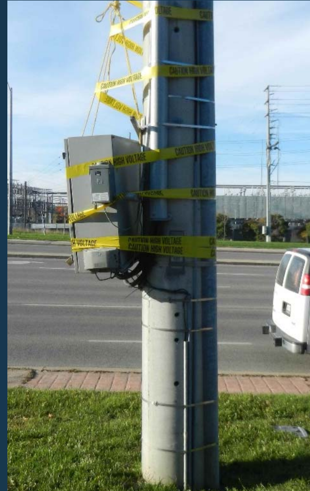
Knocked off pole by lawn tractor
