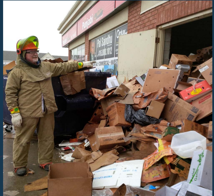
Impeded access to Elec. Rm. & Fire Hazard
